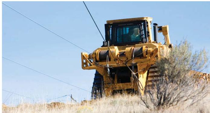
Heavy conductor and an extremely wide span contribute to very high tensions, making bulldozers the method of choice for rolling-up old conductor
