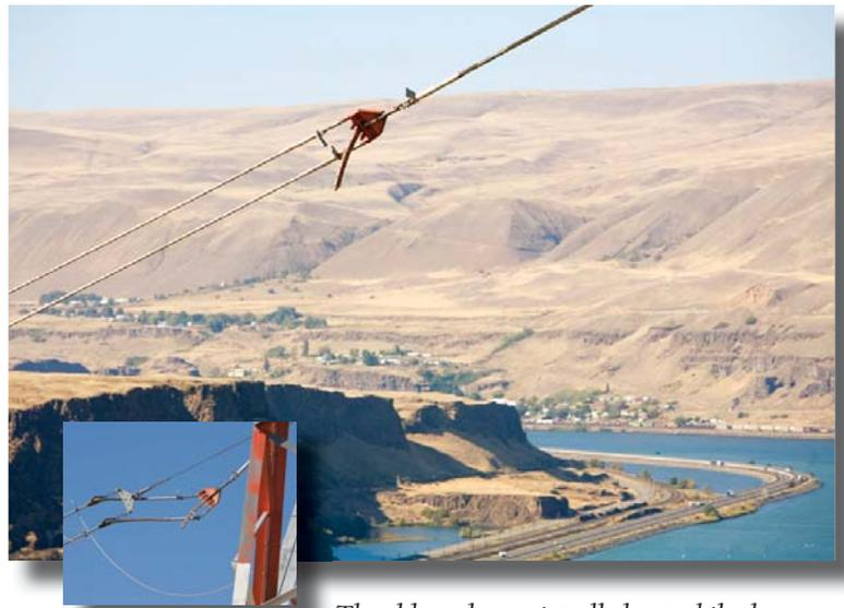
The old conductor is pulled out while the new conductor is pulled in INSET: A closer look
