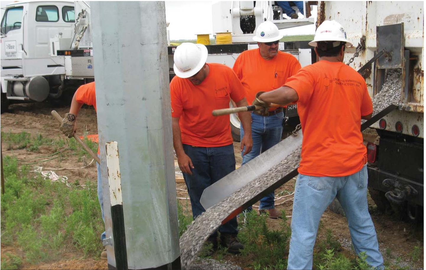
**Foundation backfilling on new transmission line structures**
