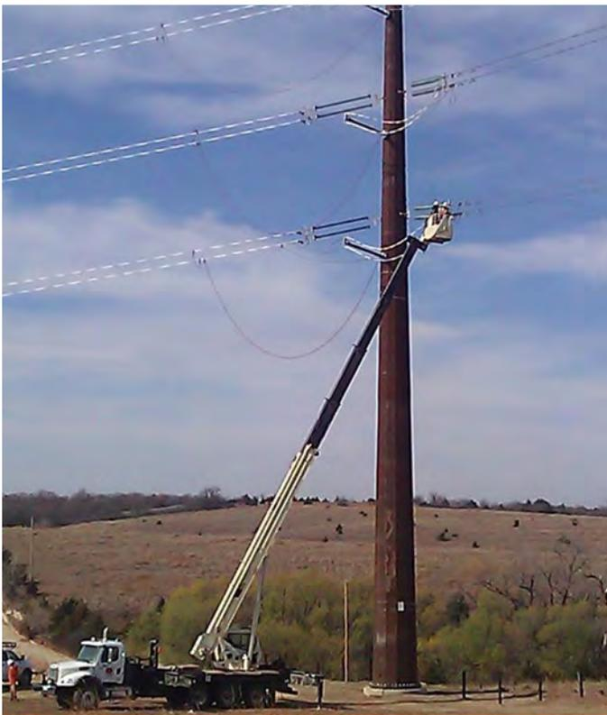
**An L.E. Myers crew installs conductor jumpers on the project’s last structure built.**
