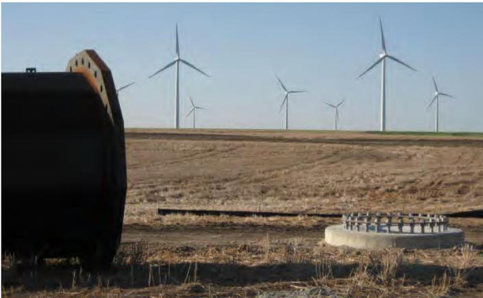
Nearly 3,000 MW of wind generation is proposed for interconnection near the new line, which was constructed primarily with singular tubular-steel poles to minimize land-use impact. Structures are 100 to 150 feet high, with an average of 900 feet between them.
