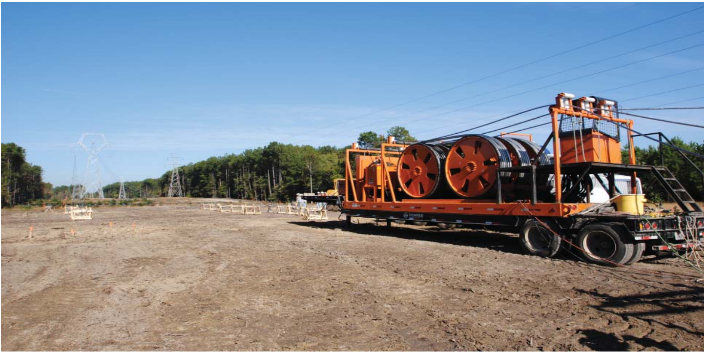
READY TO ROLL: A wire set-up on the Carson to Suffolk 500kV transmission line.
