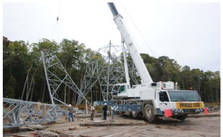
One of MYR's new 200T A T cranes helps to set one of the new lattice towers along the Carson to Suffolk 500kV transmission line.
