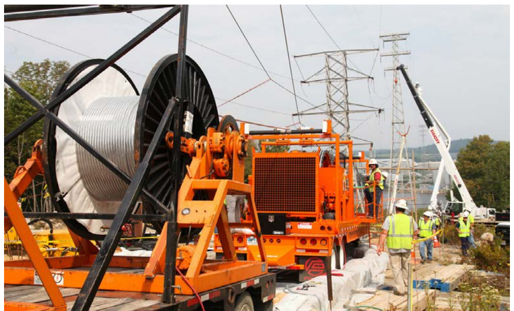
Our fleet of specialty transmission equipment delivers on challenging river crossings
