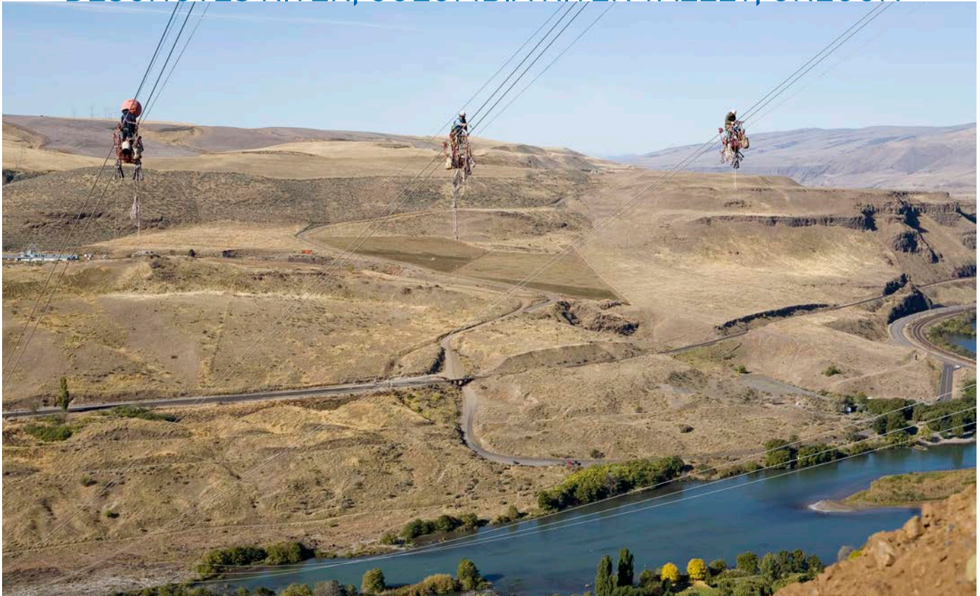
A crew installing spacers over the Deschutes River
