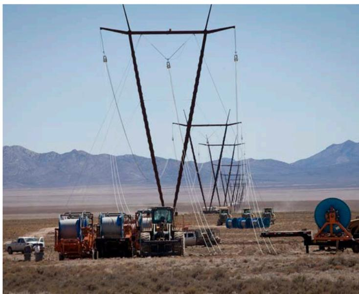
**A VERY VORACIOUS VENTURE:** Sturgeon Electric crews constructed 866 of these 146’ tubular guyed-V structures along the 235-mile route.
