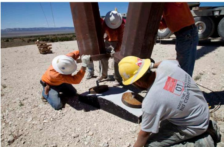
**ALL SET:** A crew sets one of the massive guayed-V structures into place on its six-foot foundation.
