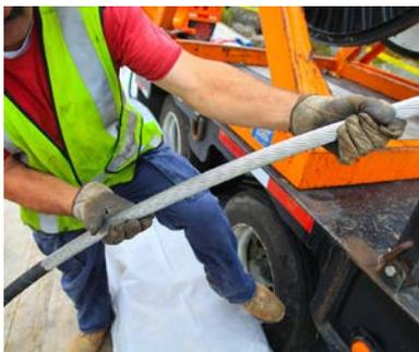
Installation of the new, high-performance ACCR conductor can run at high temperatures with low sag potential; and now allows Central Maine Power the ability to triple transmission capacity across the river.
