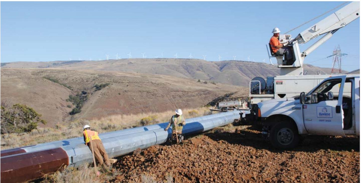
**BEAUTY IS ONLY SKIN-DEEP** - *Although numerous gorges and canyons throughout the landscape make for breathtaking views, they pose a host of challenges while constructing transmission lines throughout the area. Here, crews are assembling steel poles that make up an angle structure. The power of wind in this region is evidenced by the turbines in the background.*
